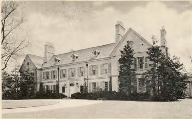
Entrance Side of Residence
